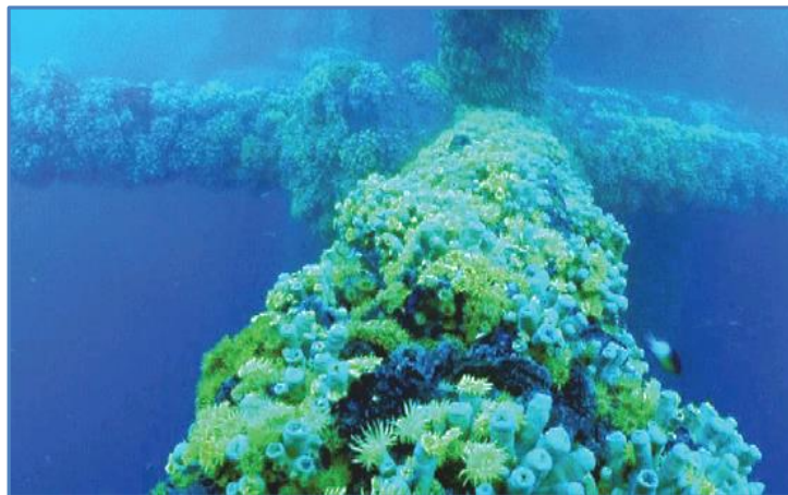
Fig. 1. Reefed jacket on the Gulf of Mexico (USA) [4]
