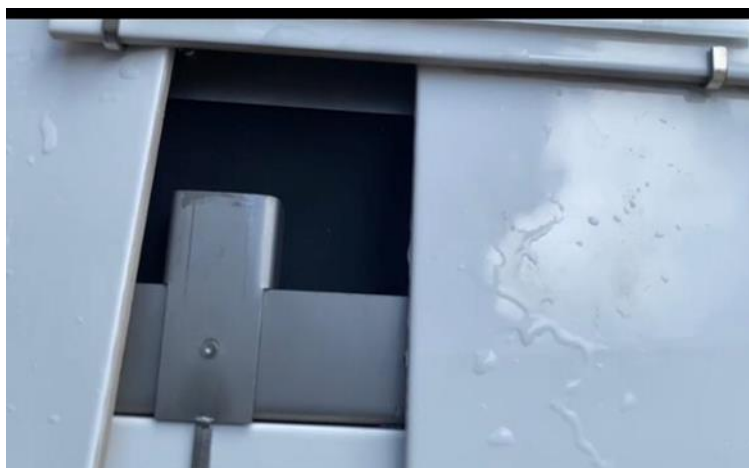
Fig. 12. Water leakage test
