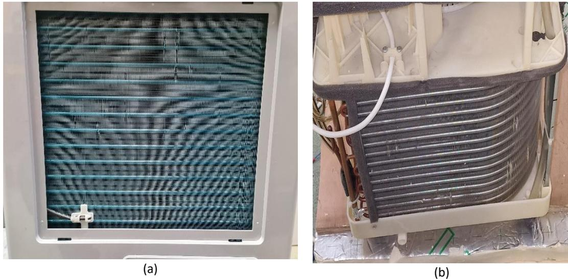
Fig. 2. Evaporator and condenser of the air conditioning system
