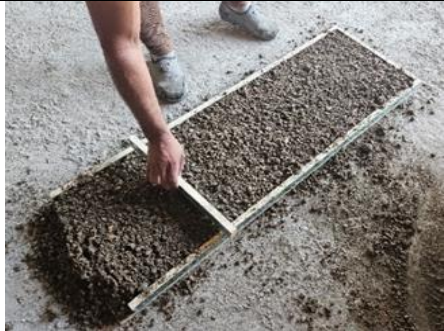
(5) Re-compacted layers to the level
