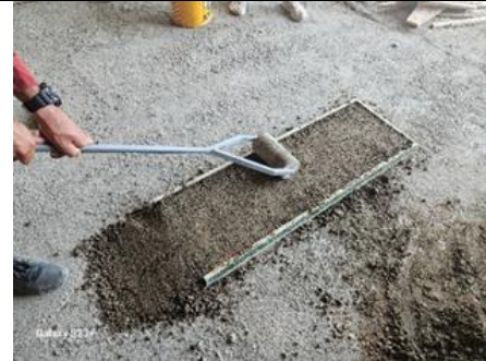
(6) levelling the surface after each layer
