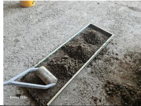
(4) Compacting in layers (3 cm)
