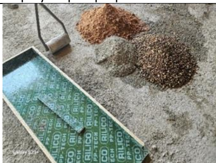
(1) Preparing the materials and mold
