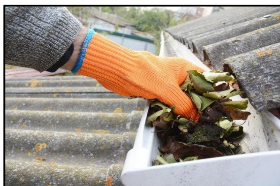
Fig. 7. Cleaning of debris
