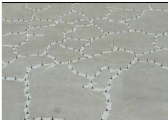
Fig. 8. Epoxy injection
