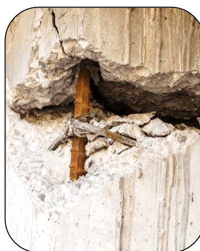
Fig. 9. Column failure
