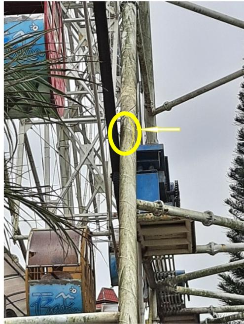
**Fig. 4.** Friction between the rim and the support pipe that causes happening scratches/flaws
