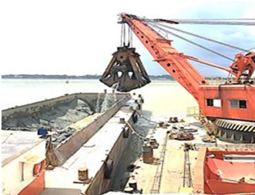
Fig. 1. Clamshell dredger (Johor, Malaysia)
