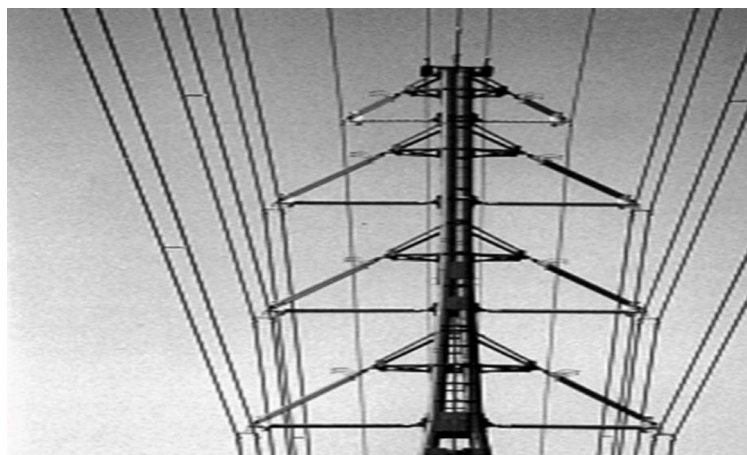
Fig. 3. Front view of a compact tower
