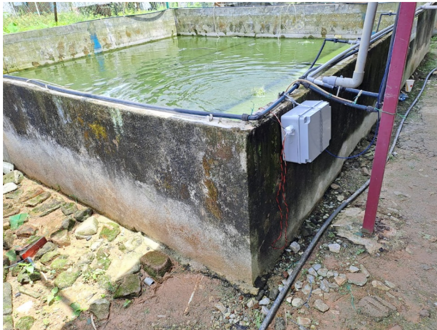
Fig. 5. Sensor node at Delek Aquaculture Farm located at Klang, Selangor, Malaysia
