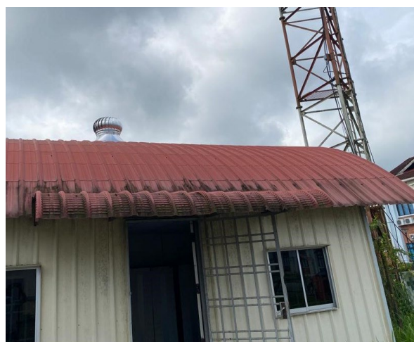
Fig. 10. Prototype development and Installation
