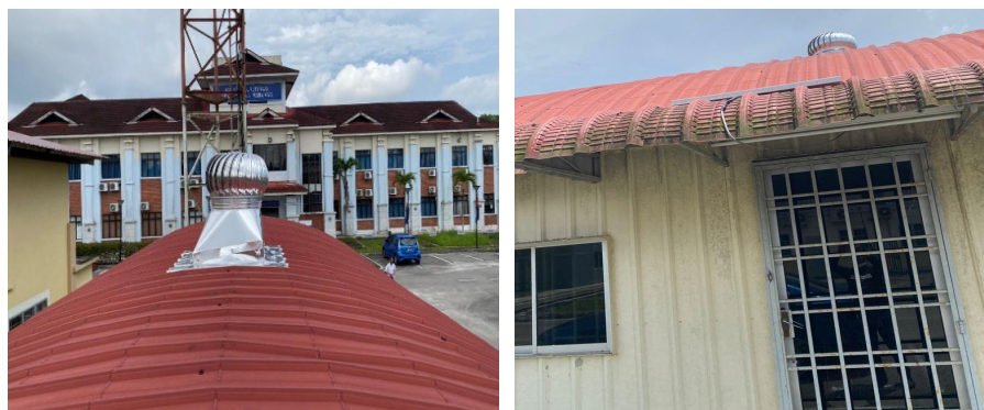
Fig. 5. Prototype development and installation
