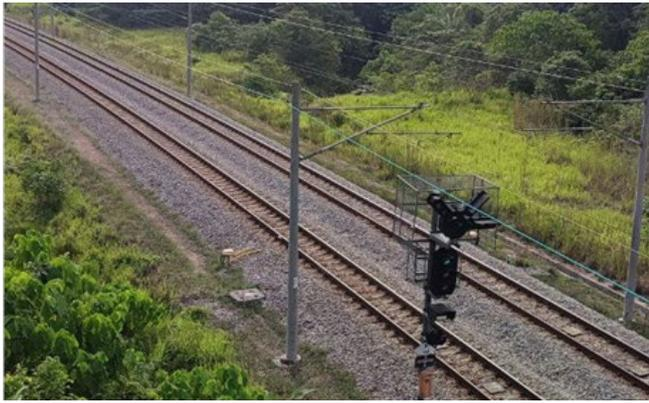
Fig. 1. Simple overhead catenary
