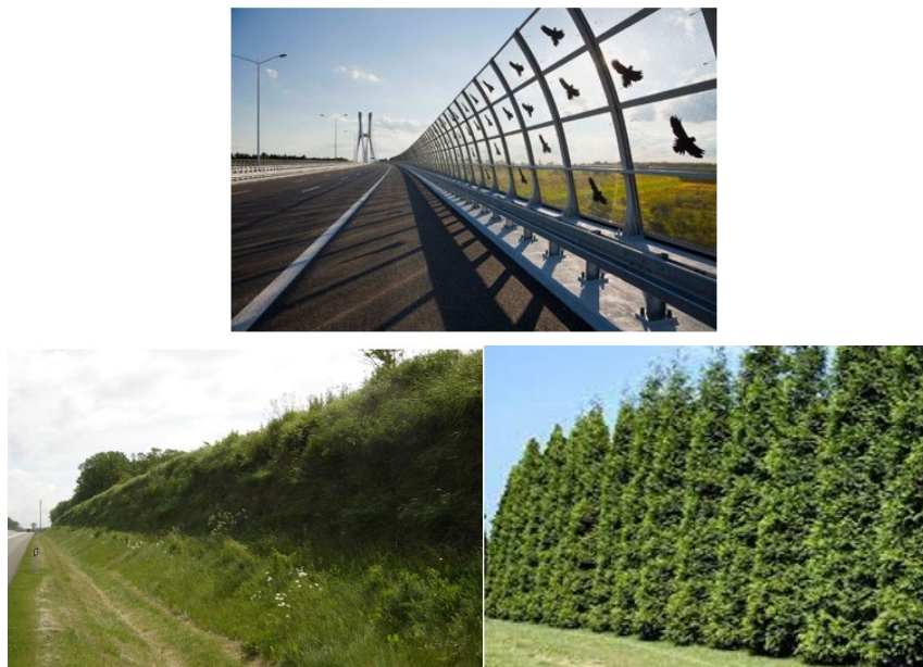
Fig. 1. Panel (top), Berm (bottom left), and Vegetation (bottom right) are the type of noise barriers
