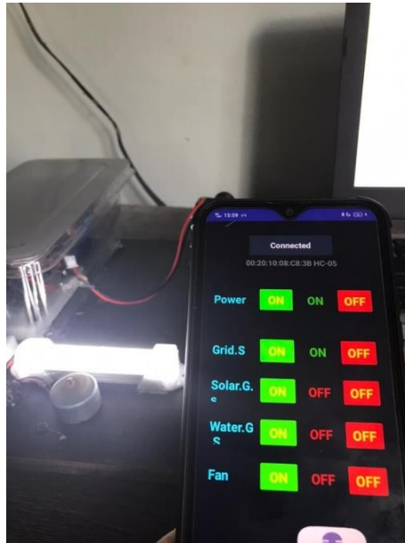
Fig. 9. Lamp and motor are turned on when switching to the grid supply
