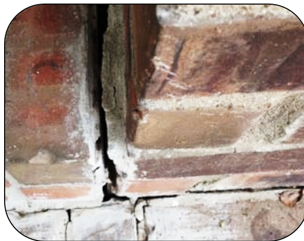
Fig. 22. Foundation cracks
