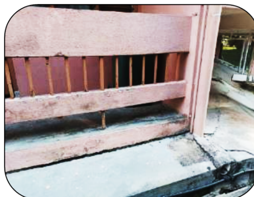
Fig. 7. Dormitory residential building
