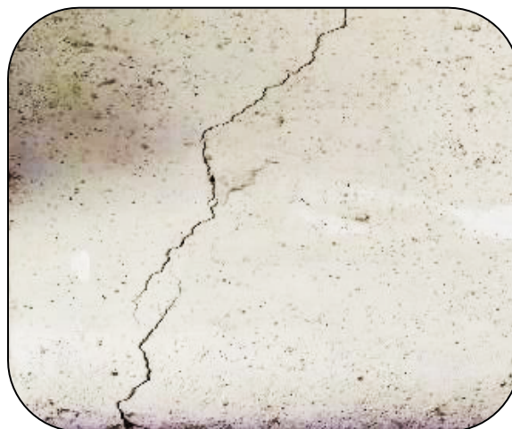
Fig. 21. Hairline cracks
