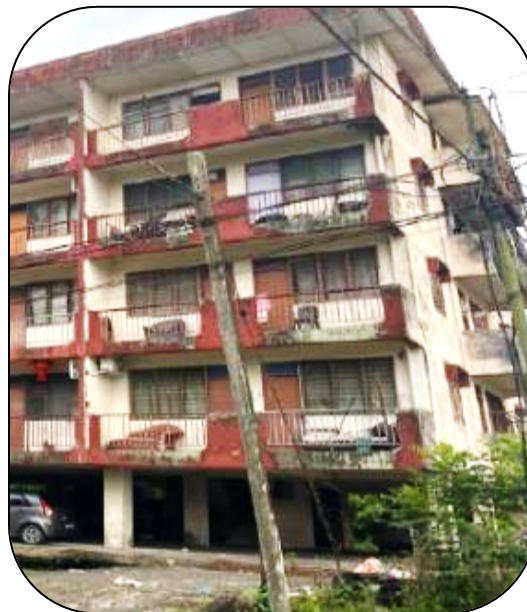
Fig. 11. External appearance of the flat
