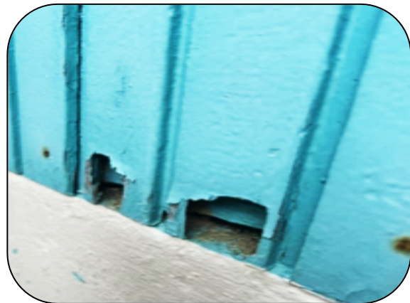
Fig. 5. Bore-holes defects
