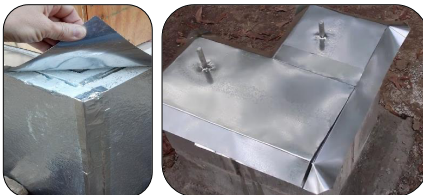
Fig. 8. Termite shields
