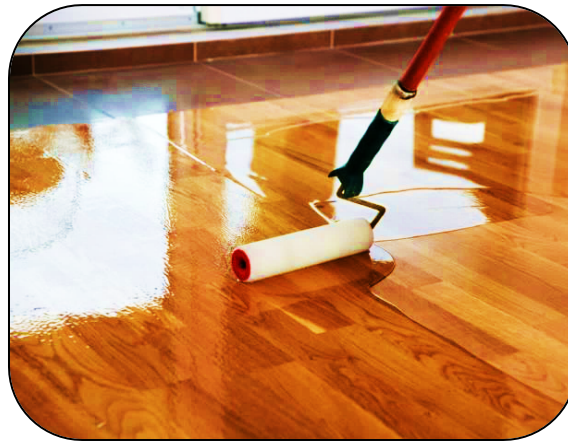
Fig. 10. Protective layer of polyurethane
