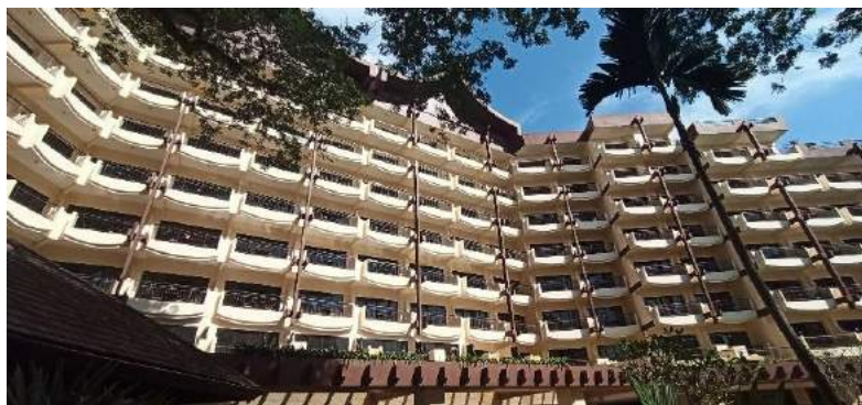
Fig. 3. Garden Wing of Shangri- La Rasa Sayang Resort
