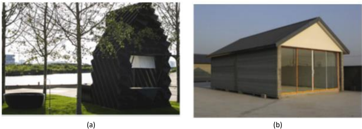
Fig. 6. a) First 3D printed house by Dus Architects b) 3D printed house by WinSun [39]
