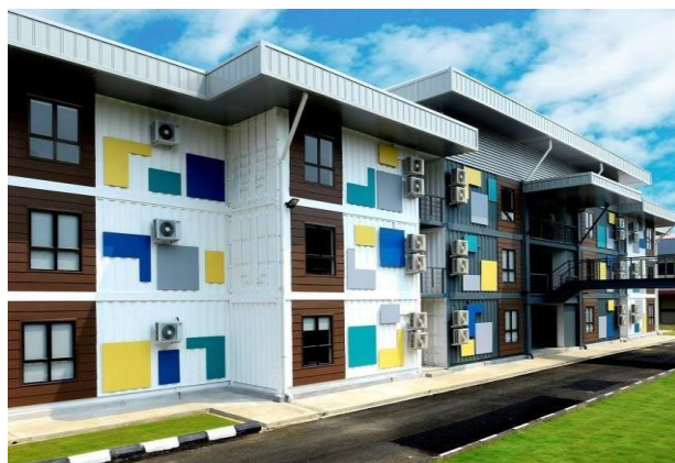
Fig. 1. 72 units of lecturer rooms in UMP, Gambang
