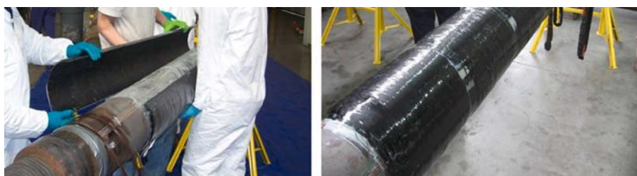
Fig. 2. Example of the process of carbon half-shells installation [10]
