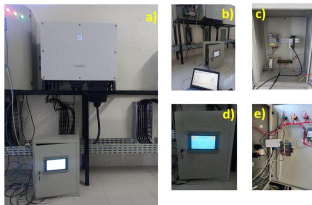
**Fig. 5.** The hardware of the monitoring system (a) Overview the System (b) PLC, HMI, and Laptop Connection (c) Wiring Installation of the system in the panel (d) Display of the HMI (e) Connection of WiFi Serial Device Server and Desktop Switch
