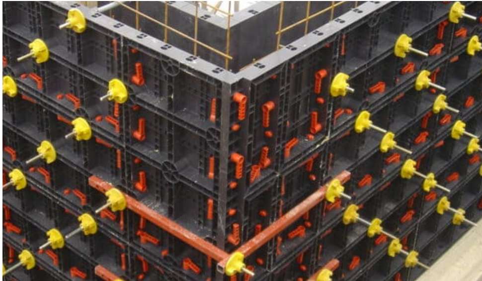
Fig. 2. Plastic formwork for concrete wall [6]
