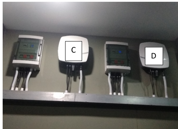
Fig. 5. PV system with uncoated rooftop
