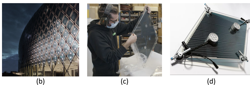
Fig. 4. Novartis Pavilion, Switzerland Organic Photovoltaic System [18]
