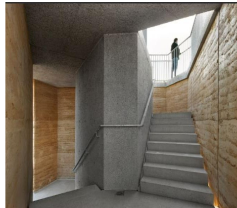
Fig. 2. The ochre-rammed earth used in constructing the external wall is reinforced with a concrete core to enhance its strength
