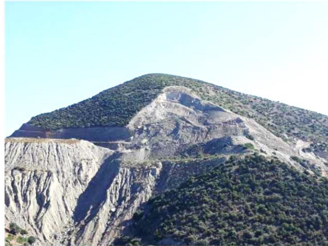
Fig. 2. Large-scale slope movement at the embankment cut on the National Road N° 16 (Jebha - Amtar)
