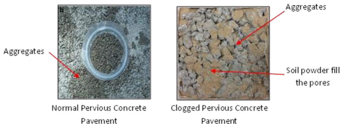
Fig. 5. Comparison of normal pervious concrete pavement and clogged pervious concrete pavement [28,30]
