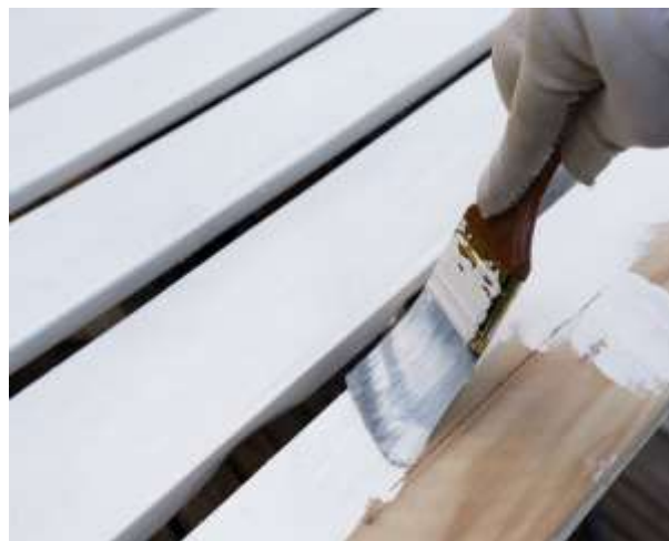
Fig. 12. Repainting decayed timber surfaces
