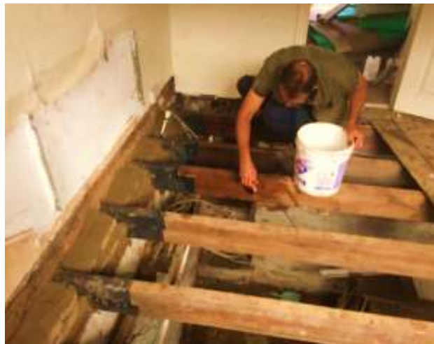
Fig. 9. Chemical agent treatment on timber surfaces
