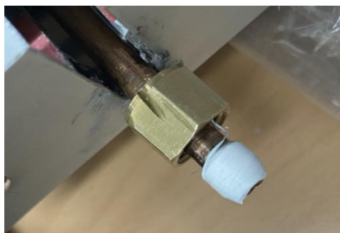
Fig. 5. Anti-leaking white tape tied on water inlet and outlet
