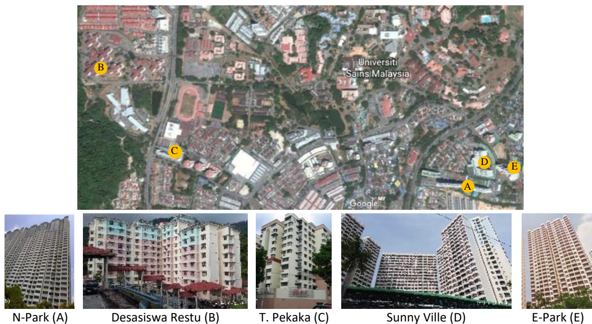
Fig. 1. Location and external view of the selected buildings for the field measurements [20]
