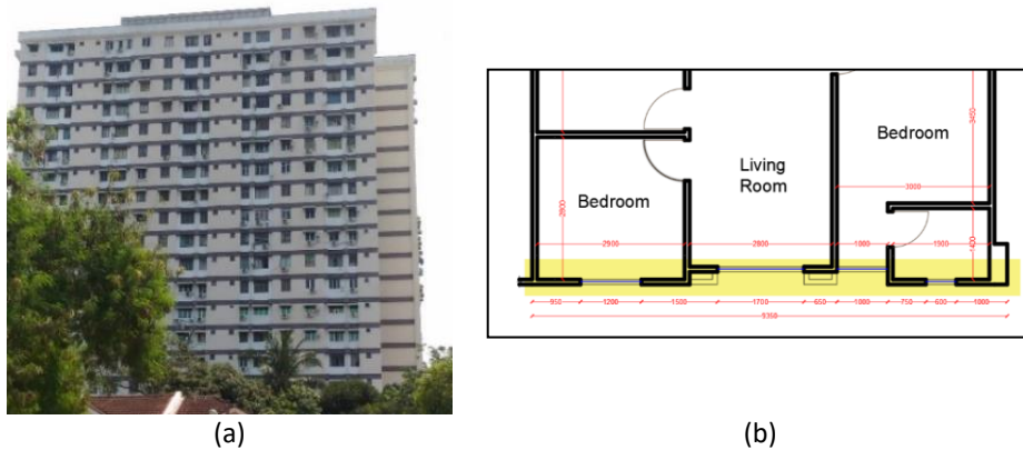
Fig. 3. Halaman Kristal 5, (a) external view and (b) the west façade of the selected apartment
