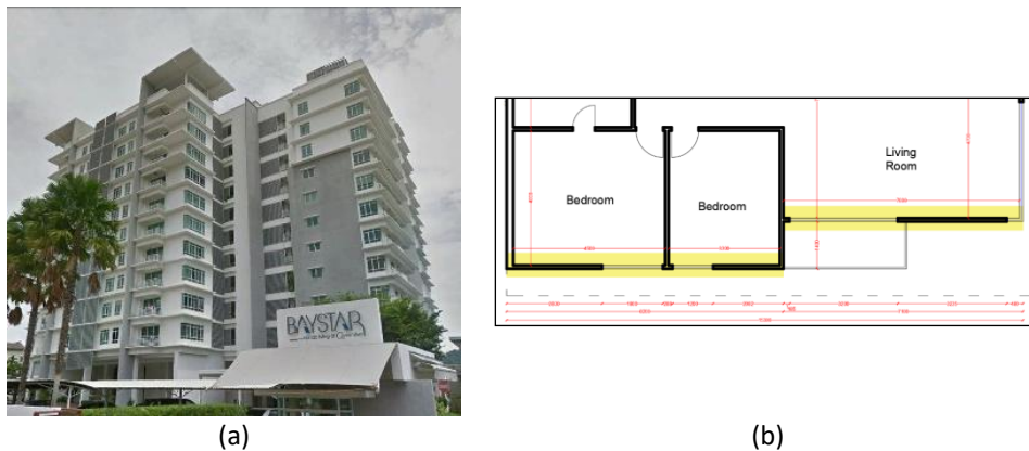
Fig. 6. Baystar, (a) external view and (b) the west façade of the selected apartment
