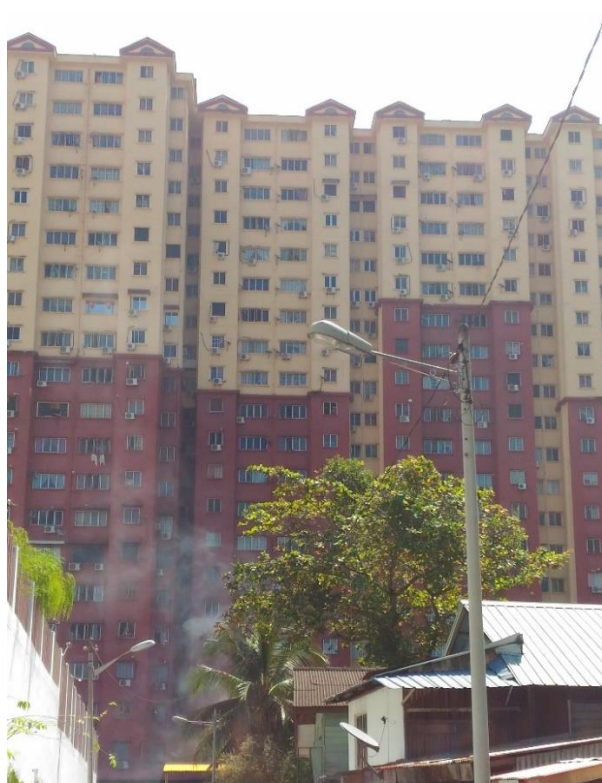
Fig. 1. Case study building; Mutiara Idaman 2
