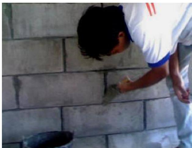
**Fig. 1.** Lightweight foamed concrete blocks being used in a housing project in Malaysia
