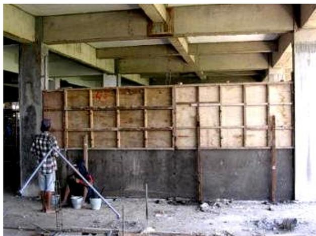
**Fig. 2.** Cast in-situ lightweight foamed concrete wall in Surabaya, Indonesia
