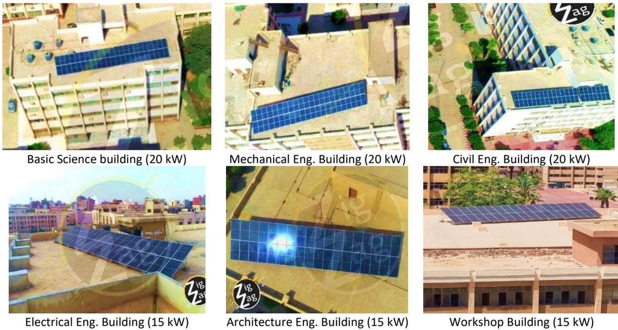
**Fig. 17.** Installed PV System on Six Buildings of the Faculty of Engineering
