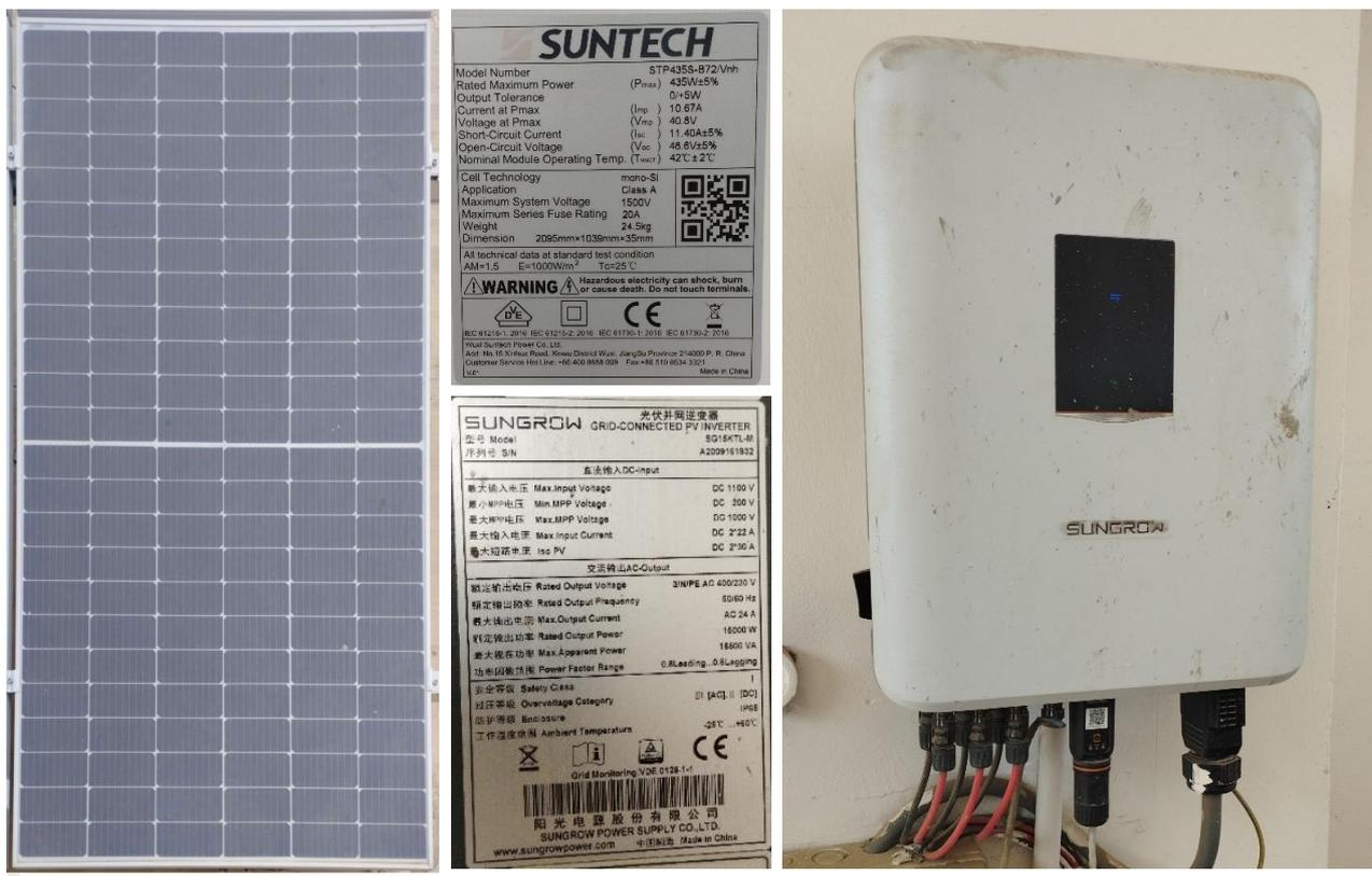
Fig. 7. Actual installed inverter and module and their nameplate
