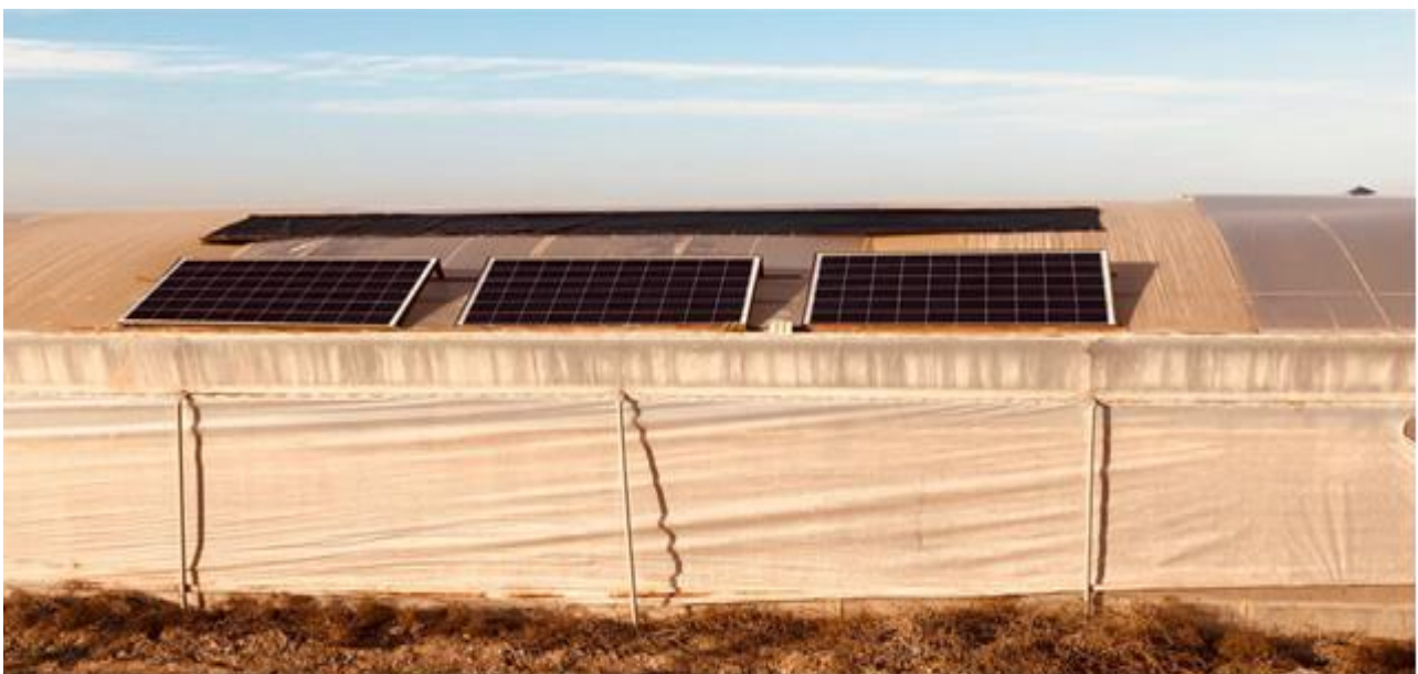
Fig. 17. The installation of solar panels on the greenhouse
