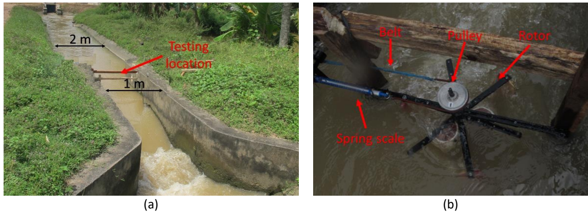
Fig. 2. Photograph of the Irrigation: (a) Rice field irrigation; (b) Turbine experimental
