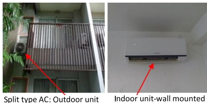
Fig. 3. Split AC system installed in residence buildings
