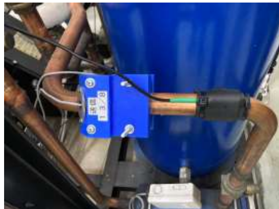
Fig. 6. Ultrasonic sensor for measuring flat gas
