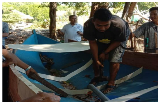
Fig. 6. Frame pattern making
