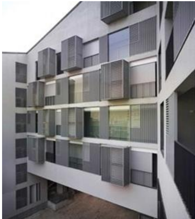
Fig. 16. Shows the overall façade after the installation of external models
