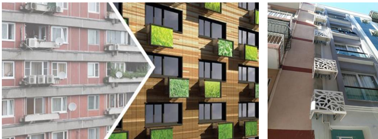
Fig. 14. Image result of before and after hiding the air conditioner in the facade
